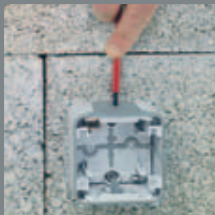
1/ Pierce the end cap using a screwdriver
