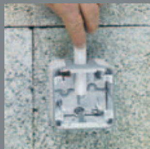
2/ Insert the tube through the end cap
