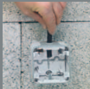
2/ Insert the cable through the end cap
